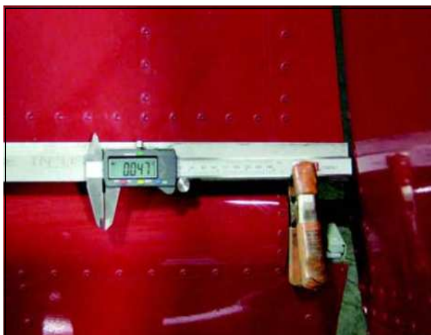
Figure 7.1: Inspect Rear Spar Doubler
